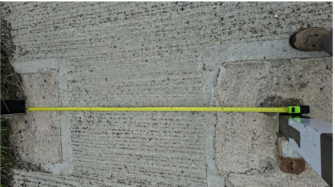
OCC TRO bollards on the Icknield Greenway, Ginge Road, East Ginge gap 1.8m
